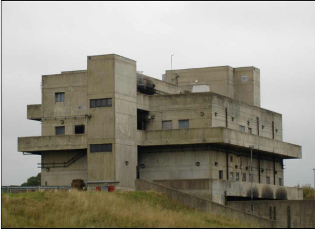
Figure 16. Large Masonry Burn Building, British Fire Service College
